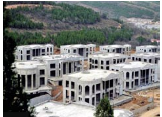
But where is Capability Brown'. Where the unmown grass lapping the ruined rustications? Where the dreamy evocation of Claude Lorraine? This is like those courtyards filled with the broken busts of Lenin and Stalin after Glasnost. It Is not even a 'street'.
